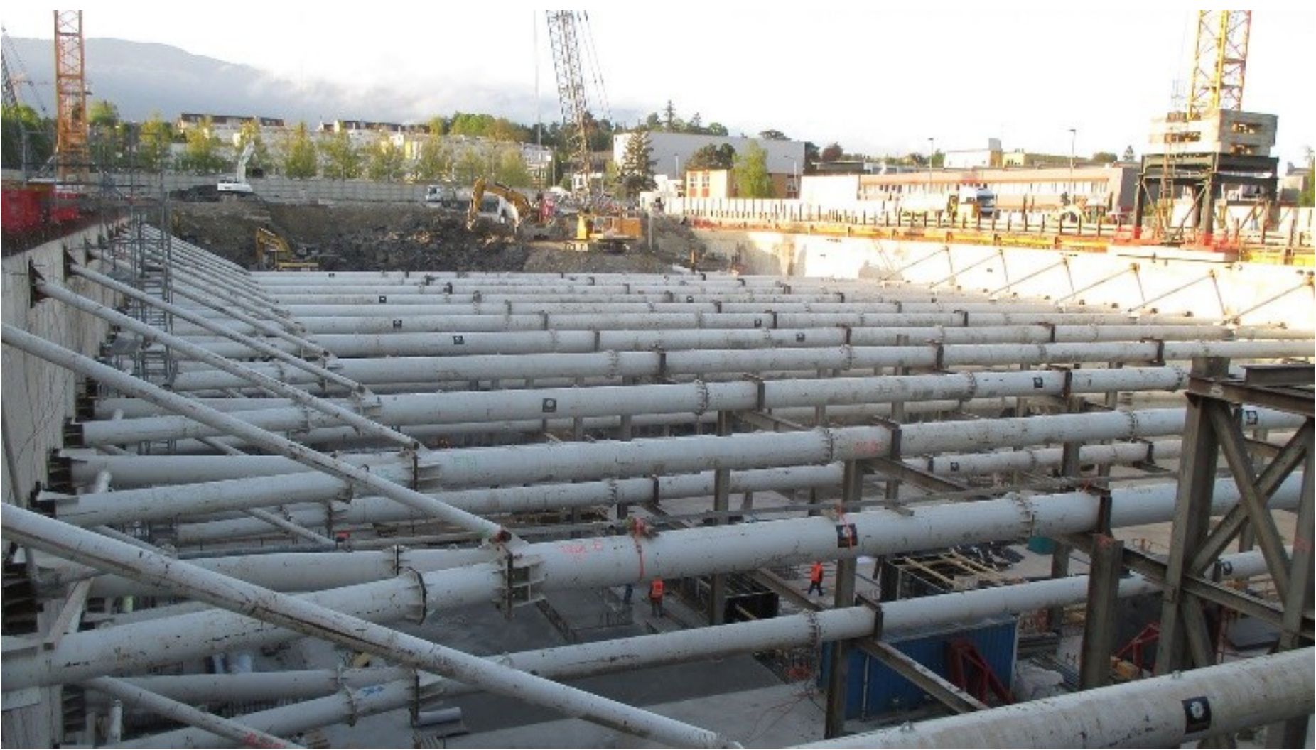
Typical braced excavation, Geneva, 3 levels of struts
