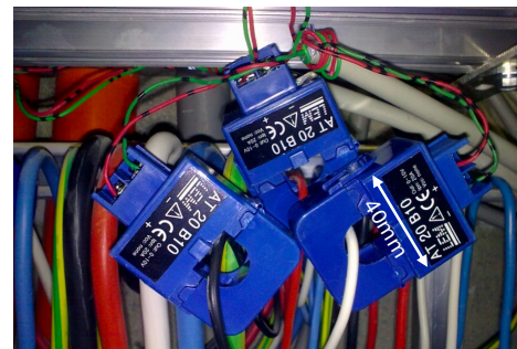
Fig. 2. Hall sensors on Building D Light.
